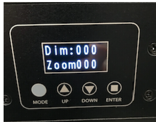
NO DMX CABLE CONNECTED
